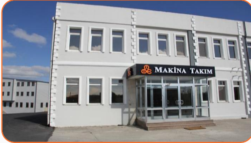
Production Facility / Factory Headquarters
